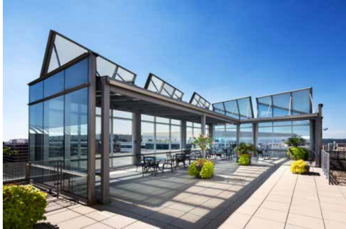
EXISTING PENTHOUSE ARCHITECTURAL EMBELLISHMENT AT PENNSYLVANIA AVENUE AND 19TH STREET NW
