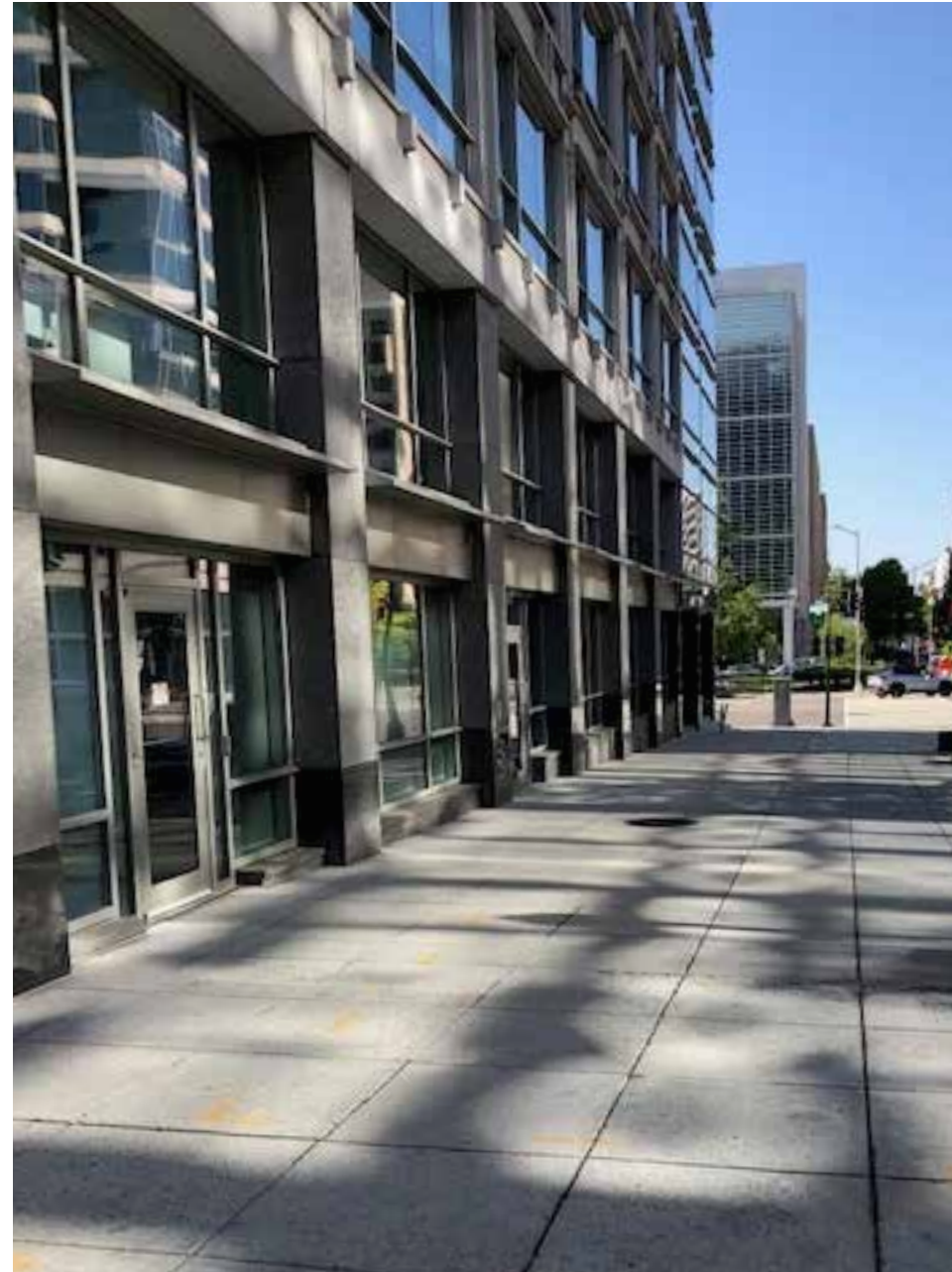
EXISTING BUILDING 19TH STREET NW LOOKING SOUTH
