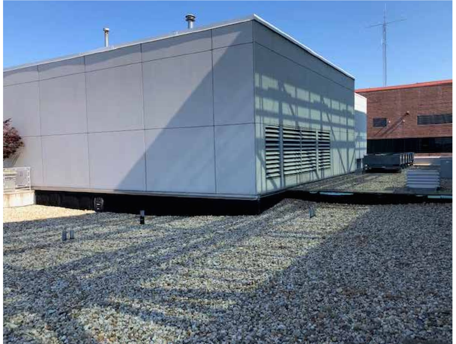
EXISTING PENTHOUSE SOUTHEAST CORNER LOOKING NORTHWEST
