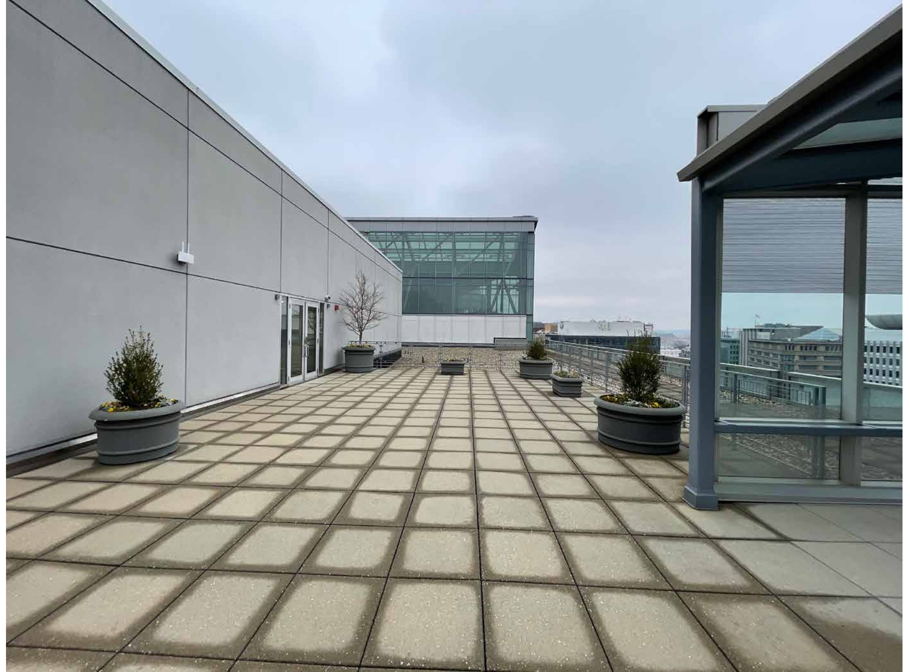
EXISTING PENTHOUSE SOUTH ELEVATION WITH EXISTING EMBELLISHMENT (RIGHT SIDE OF IMAGE) (1875 PENNSYLVANIA AVENUE NW BEYOND)
